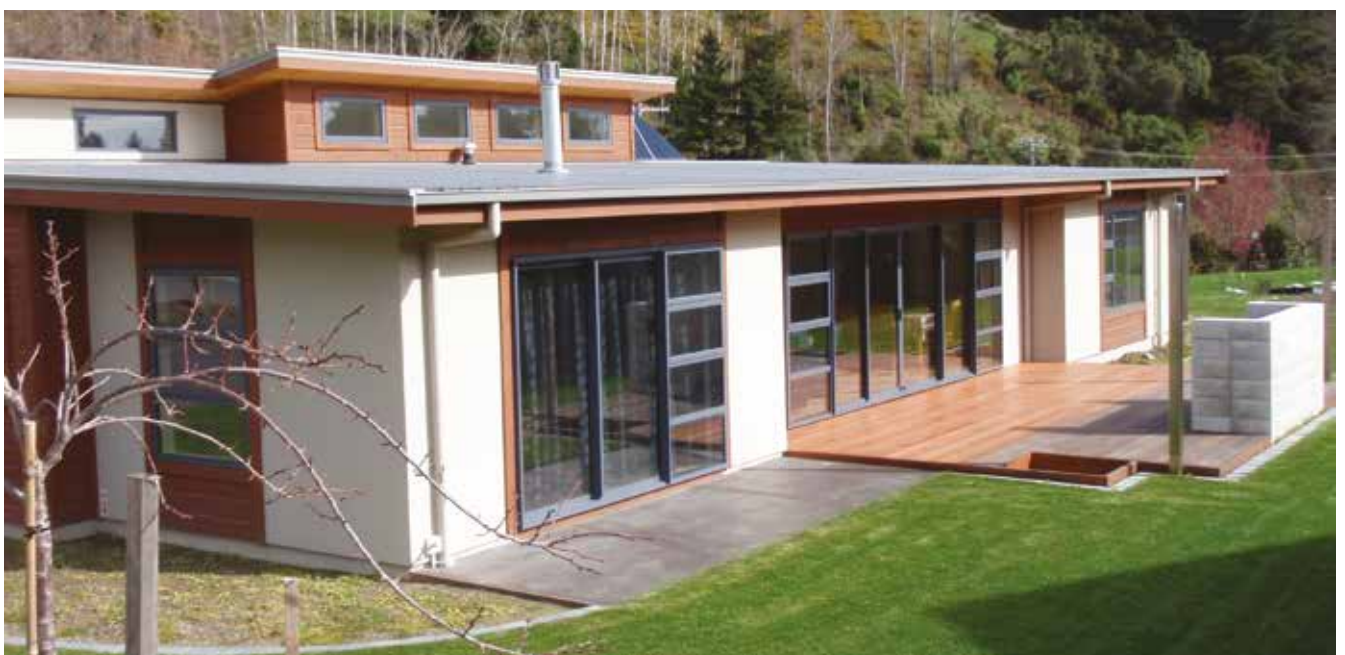
Above: North-facing full-height glazing with eave design admitting all winter sunshine – plus clerestory windows, also with eave control, admitting full winter sunshine to rear interior spaces.
