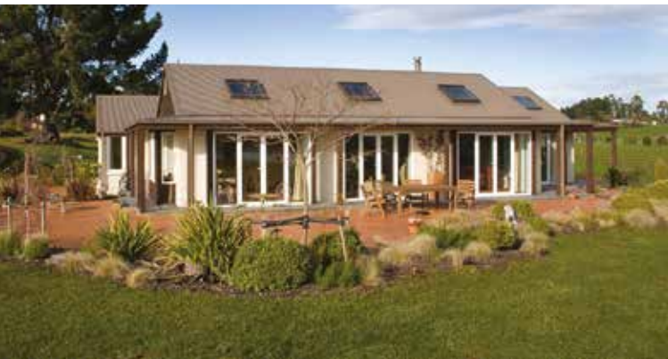
Above: This house makes the most of full sun on the north glazing, with veranda awnings to control the sun in summer. Skylight windows admit light into the airy interior. Photos: Mark Fielding
