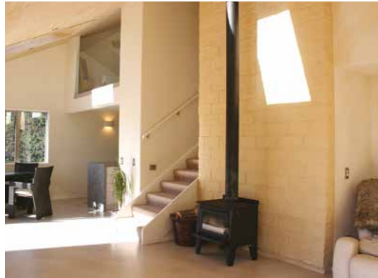
Above: Interior main space in the Cooke house at midday in mid-winter: solar gain through full-height north glazing irradiating thermal mass floor, with north-facing skylights irradiating the adobe thermal mass wall. The small radiant log burner is used for backup heating only.
