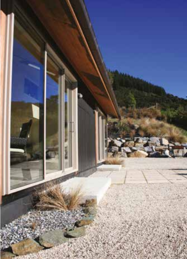
Above: The Cooke house: Eave design that allows all available winter sunshine to enter through full-height north glazing. Photos: Mark Fielding
