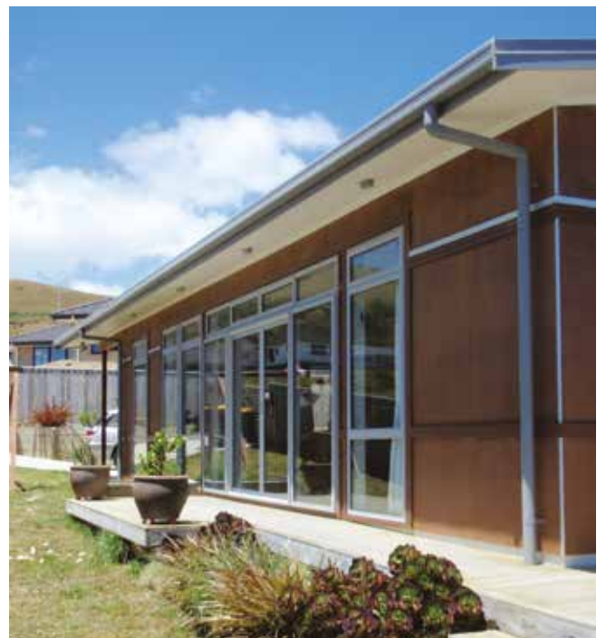
Above: The Lewis house, Tawa. A compact, affordable house using passive solar design. This photo shows the sunshine angle on the longest day, with eaves completely controlling solar admittance.
