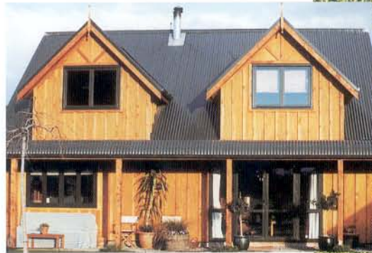
Below Traditional board and batten is created using AlpineClad Type 3000 with battens overlaid at set spacings.
