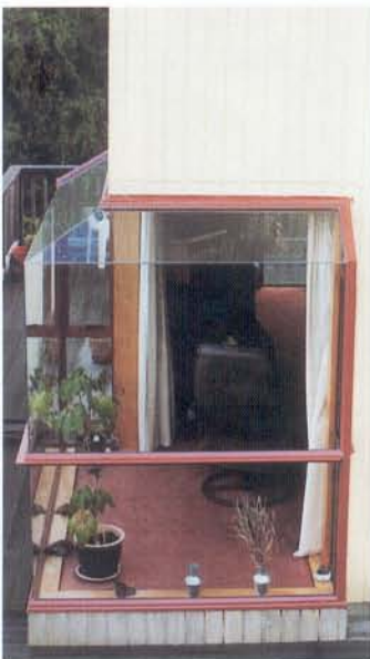
Above and right This accommodation block is constructed with AlpineClad Type 3000 with battens overlaid.
