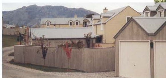
Above Millbrook Resort showing AlpineClad 1000/100 Left AlpineClad Type 1000/100 combines with unusual bay window for modern effect.
