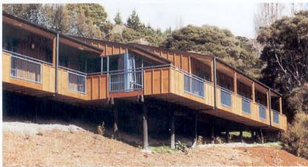
Above and right This accommodation block is constructed with AlpineClad Type 3000 with battens overlaid.
